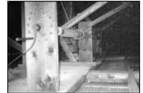
The North Dartmouth Meeting House's overhead pulley system to raise and lower the panels dividing the men's monthly meeting from the women's.
